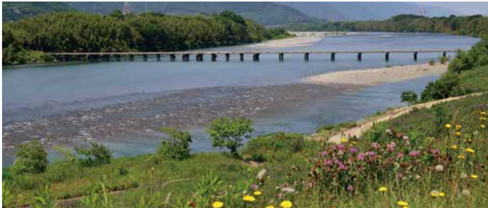
The Yoshino River The photo shows a landscape seen in Mima-shi. During floods caused by typhoons, etc., the submerged bridge is hidden in the muddy water, showing the power of the violent Yoshino River during a flood.
